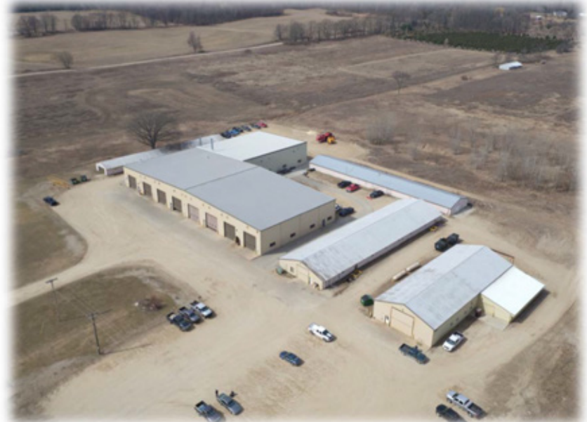
Bandit's North Winn Facility
