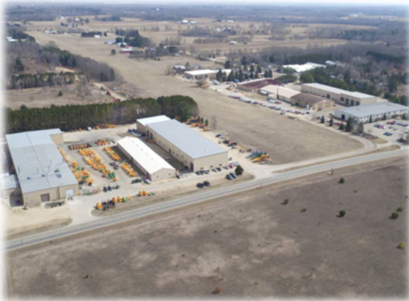
Bandit's Main Plant
